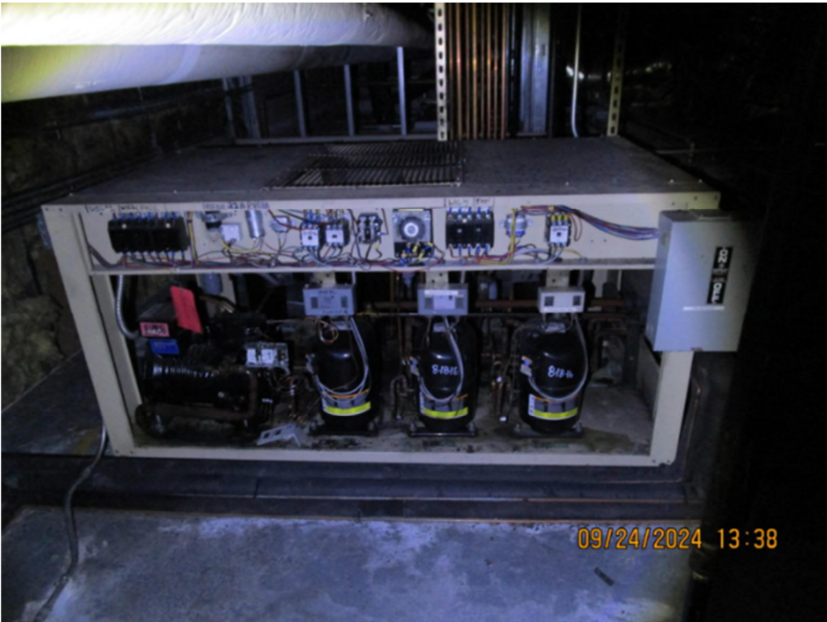
Existing compressor rack on top of the walk-ins:
